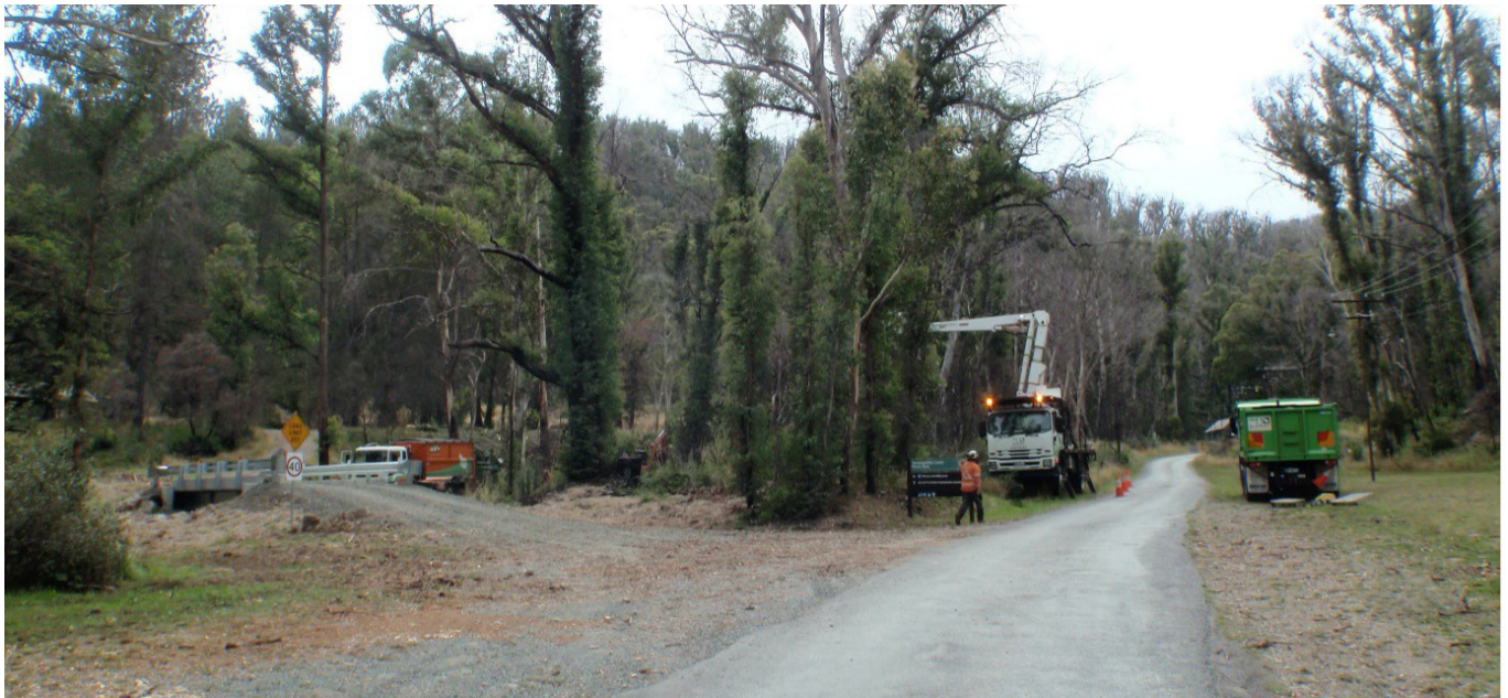
Stage 2 - Clearing of dangerous burnt trees. Stage 1 focused on creating access to Yarrangobilly Caves. The new bridge has been constructed. It provides access to the picnic areas and is higher, wider, and fireproof. The previous bridge burnt in the fire.
